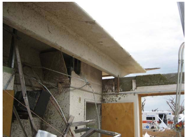
Figure 6: Hospital with Precast Concrete Twin Tees
